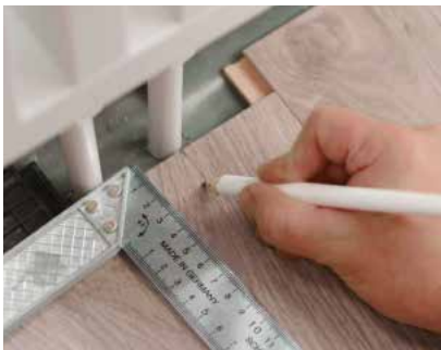
Door frame and radiator pipes
